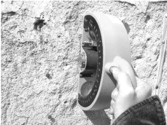
Fig. 3 Test with Schmidt impact hammer on ancient lime mortar.
