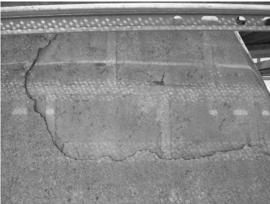
Fig. 6 The previous decorated render discovered under the layers of non decorated recovering render.
