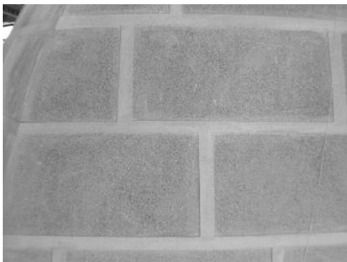
Fig. 24 Surfaces details after integration of the lacunas.
