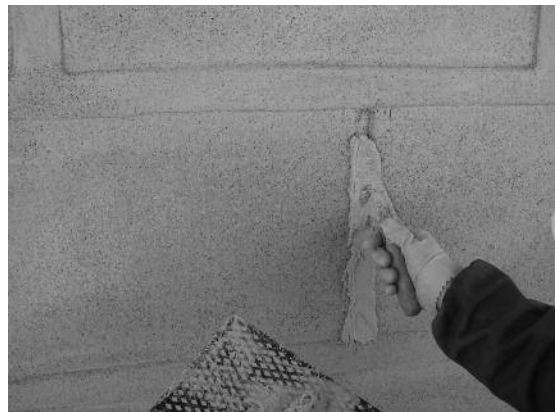
Fig. 20 Application of the mortar in the joint area.
