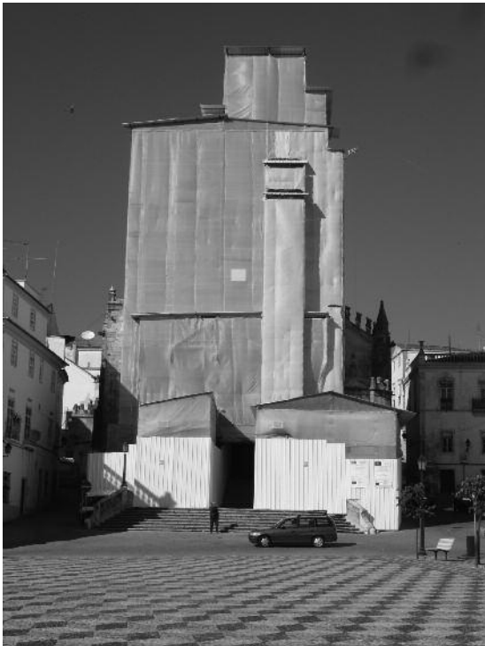
Fig. 2 Church of Nossa Senhora da Assunção during the works of conservation.
