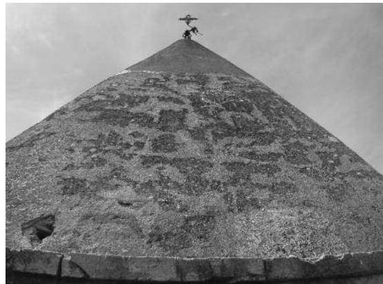
Fig. 4 Detail of the initial state of conservation.
