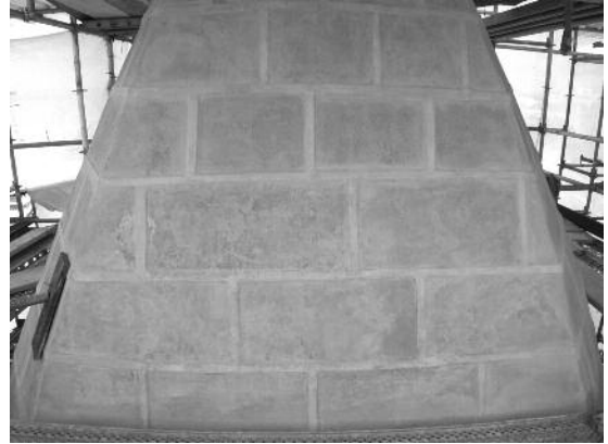
Fig. 25 Architectural surface after the integration of the lacunas.
